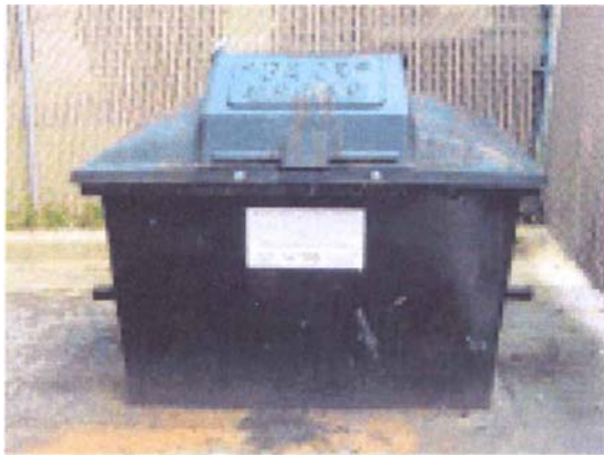
Waste grease bin (WGB)
